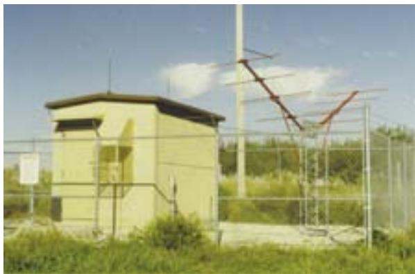
“V” shaped antennas at many longwave sites are for a separate 75 MHz marker beacon. This is LH/334 kHz, Bloomington, IL.
